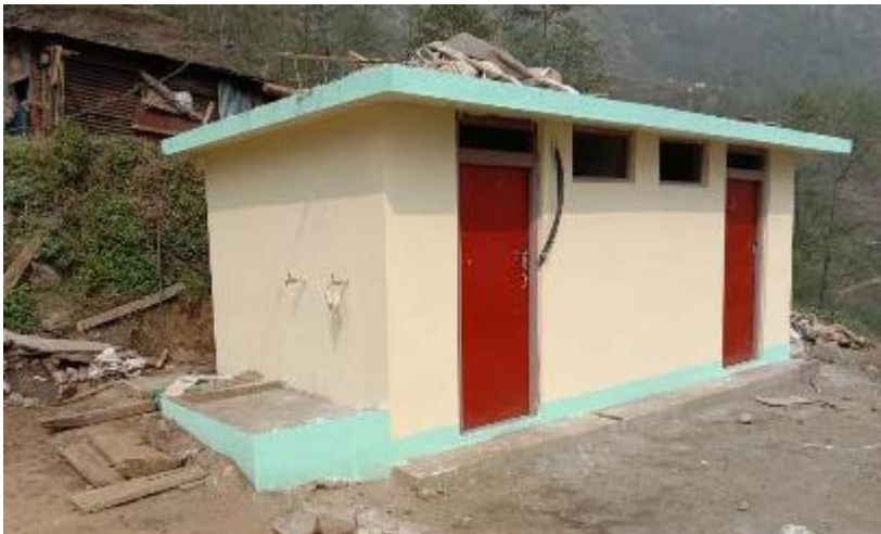
Figure 37 newly constructed double compartment toilet at Duguna
