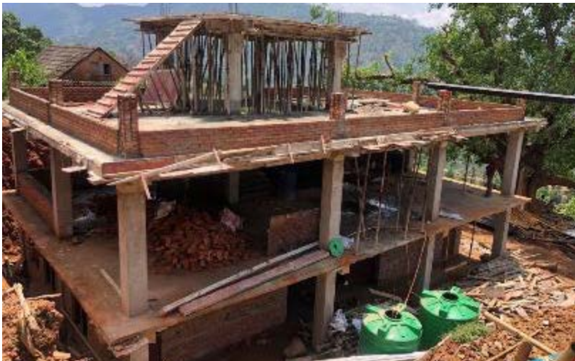
Figure 30 Janajagan BS under construction
