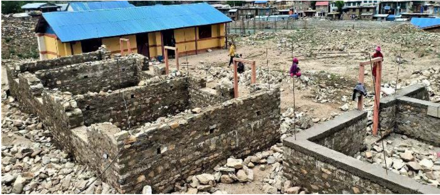
Figure 29 School building under construction in Dolpa
