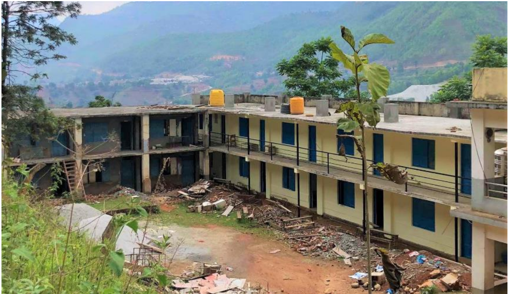
Figure 28 BLOCK A and BLOCK B of Indrawati SS at a glance
