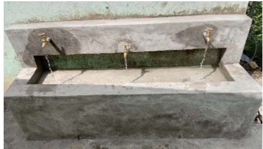
Figure 38 Taps construction at school of Bokchen
