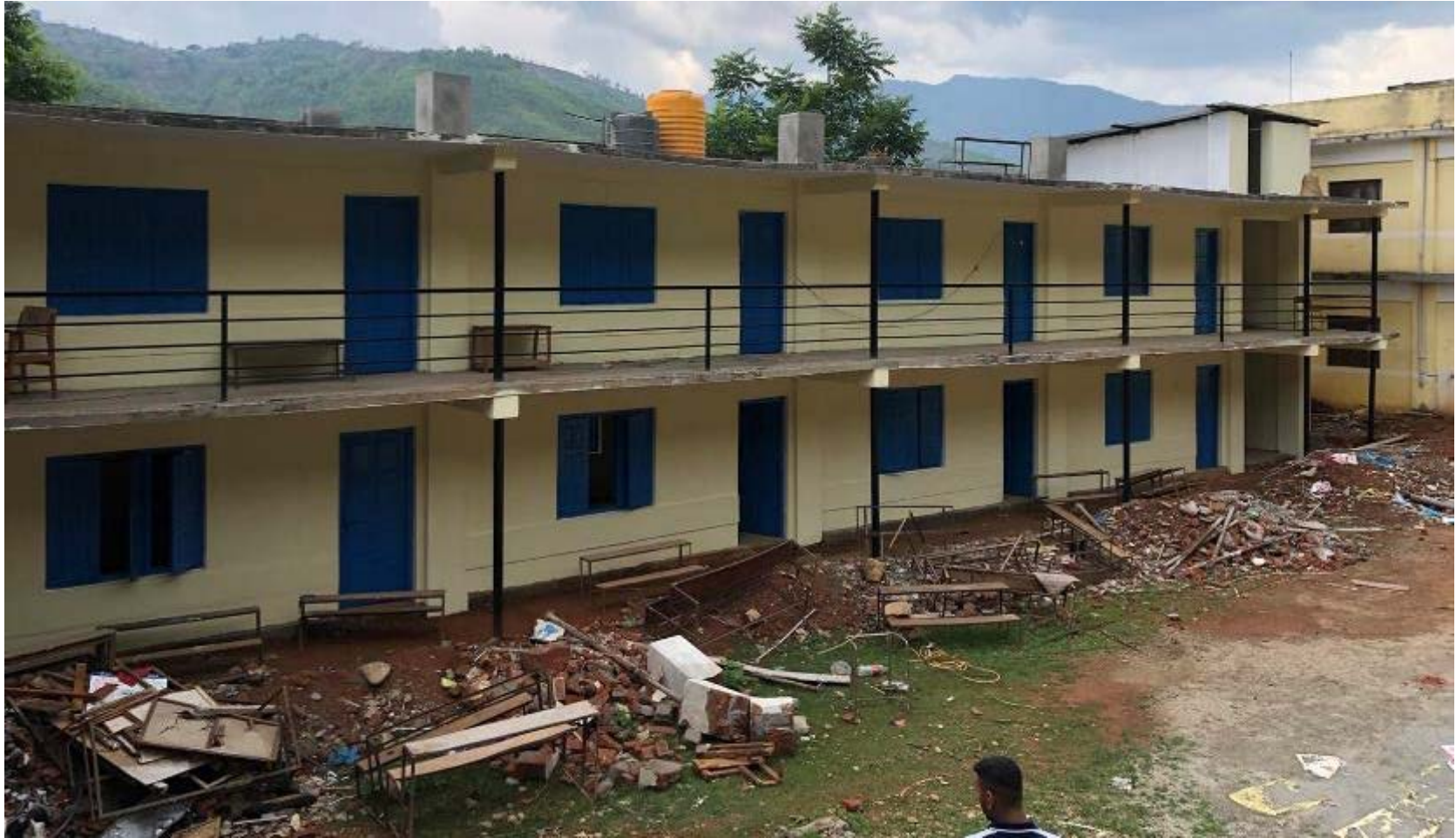
Figure 27 Indrawati Secondary School BLOCK A after retrofitting
