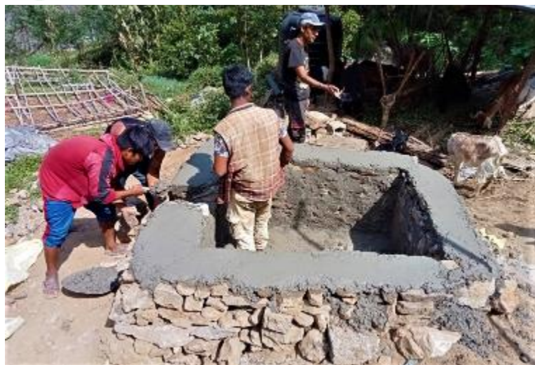
Figure 31 Biogas plant construction in Duguna
