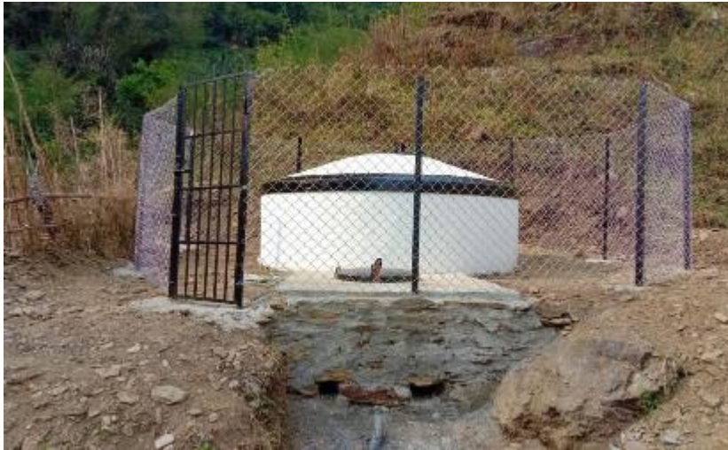
Figure 35 Reservoir Tank constructed in Bokchen
