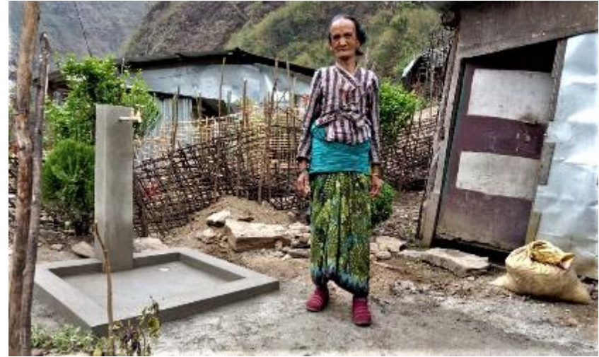
Figure 36 Taps construction completed in Bokchen
