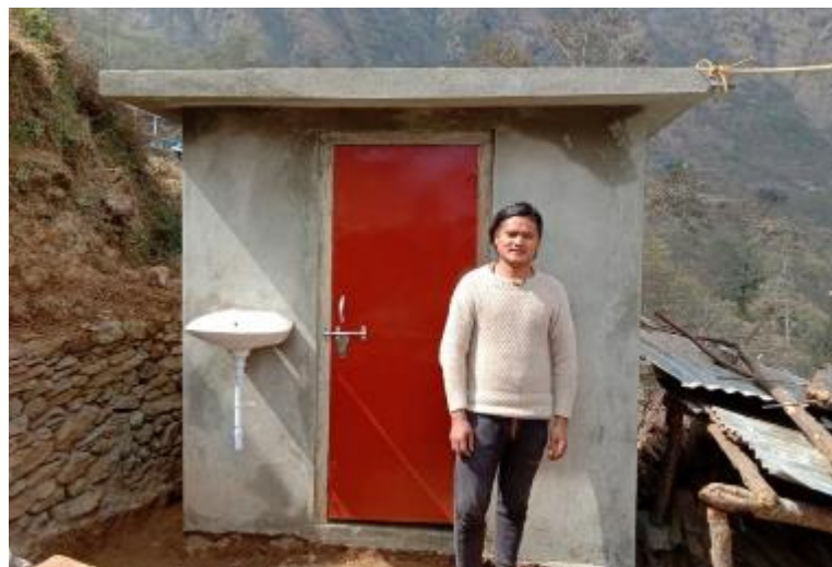
Figure 32 Single compartment with handwashing facility
